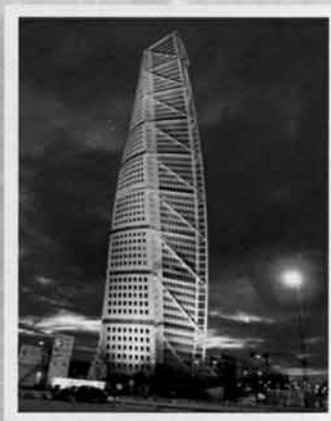
Turning Torso, a 190 m tall building for residents. Photo: Pierre Mens
